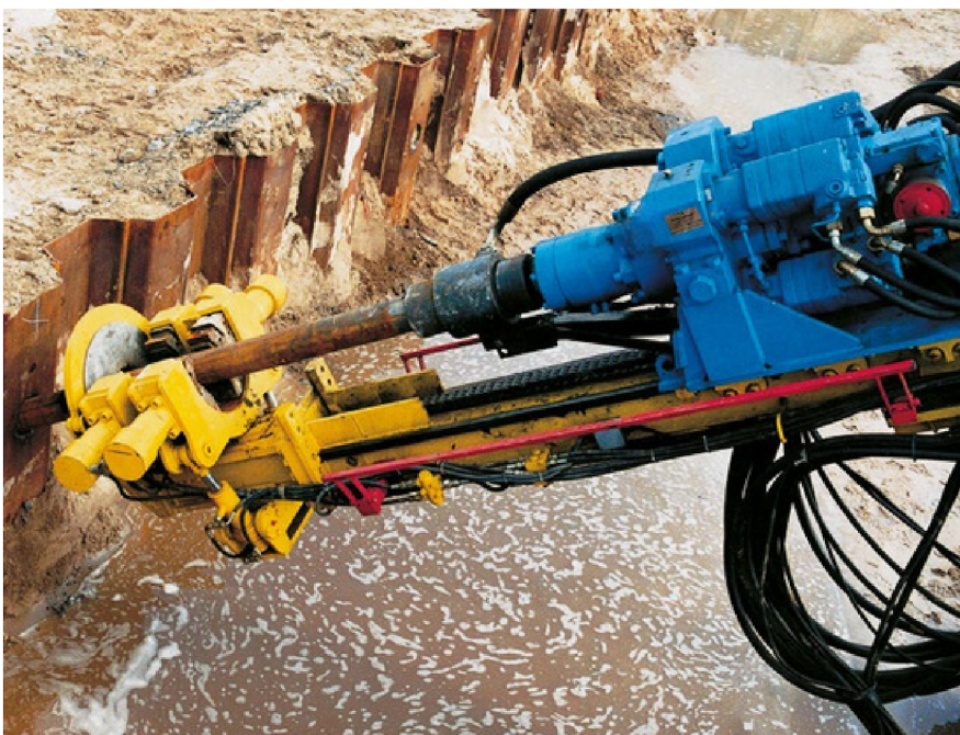
HB60 drilling 177.8 mm casings 23 m deep
