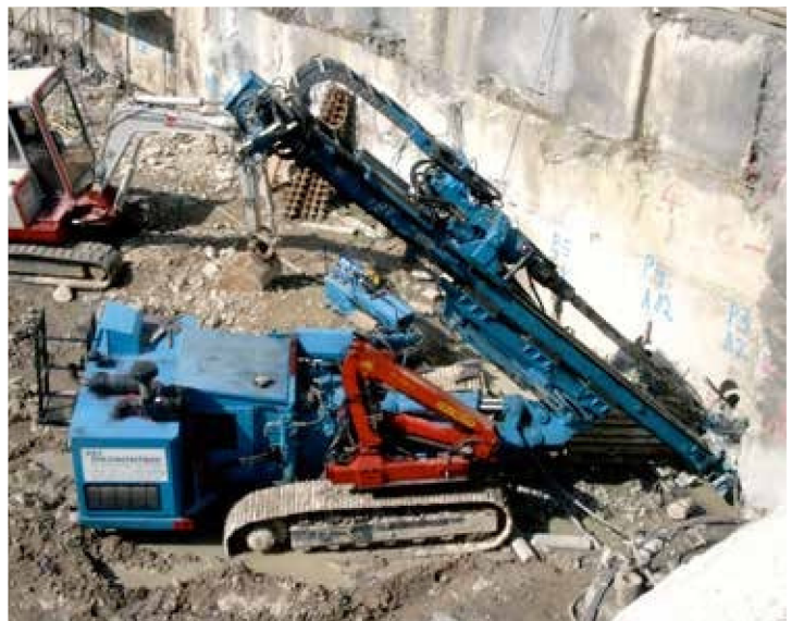
HB50 drilling 152.4 mm casings 25 m deep for strand anchors
