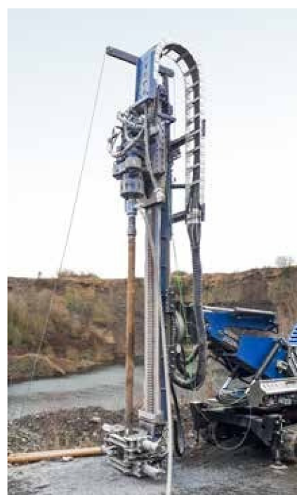
HB48 drilling in a basalt quarry
