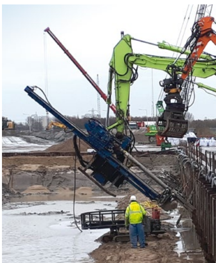
Drilling 178mm casings and 60 m long beneath excavator in sand and gravel
