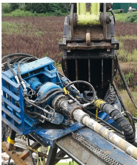
Drilling overhead 178mm casings, 48 m deep with one time drill bit
